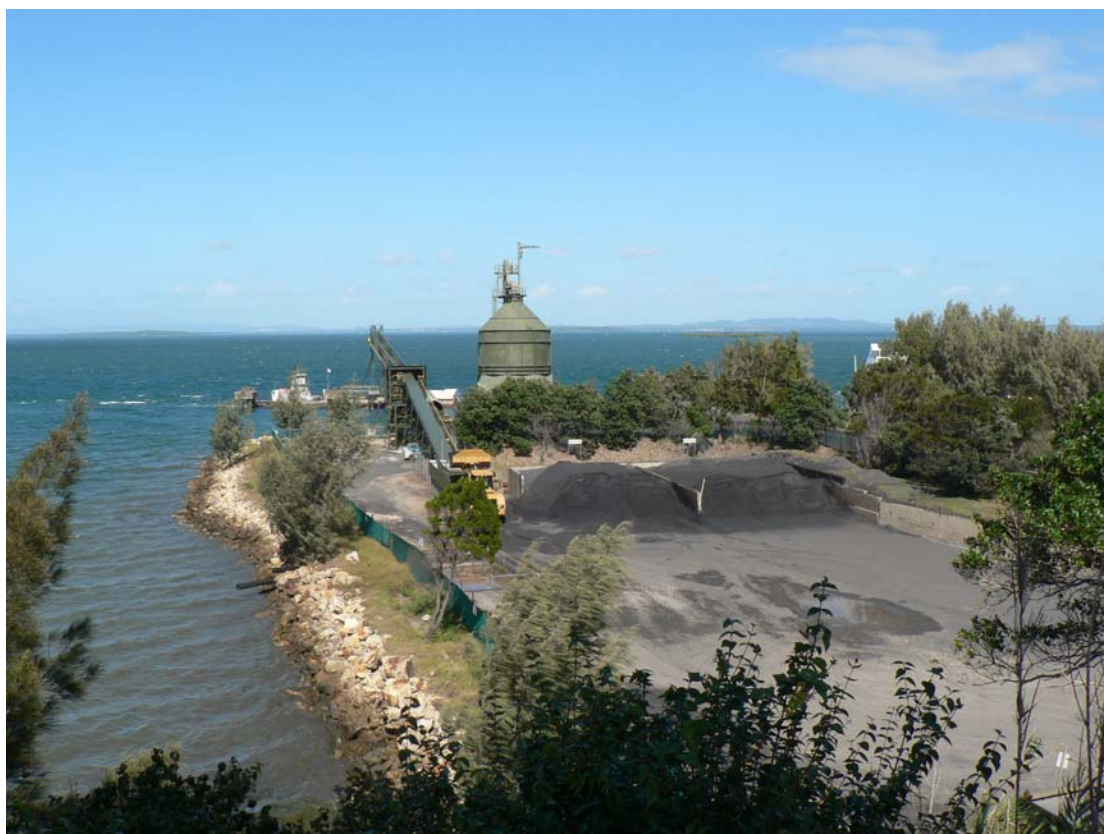
Photograph 1: View of Barge-loading Facility from Logan Crescent
